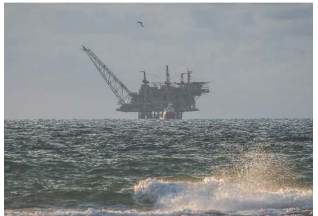
View of the Israeli Leviathan gas field gas processing rig. | Photo: Flash90
