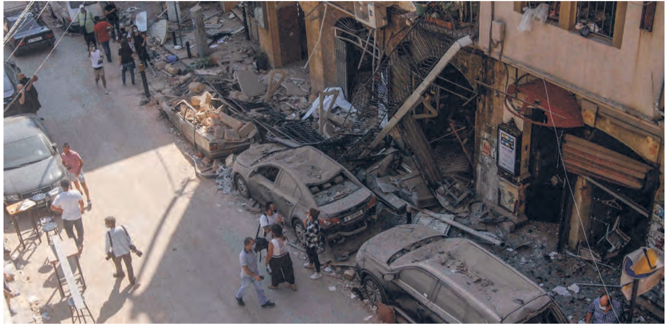
A view of damaged buildings after massive explosion in Beirut on 4 August 2020. | Photo: Flash 90
