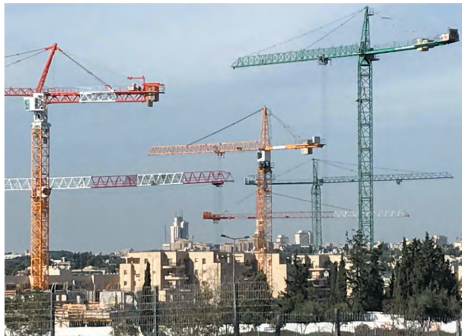
Construction taking place in Jerusalem, November 2018. | Photo: Nigel Woodley
