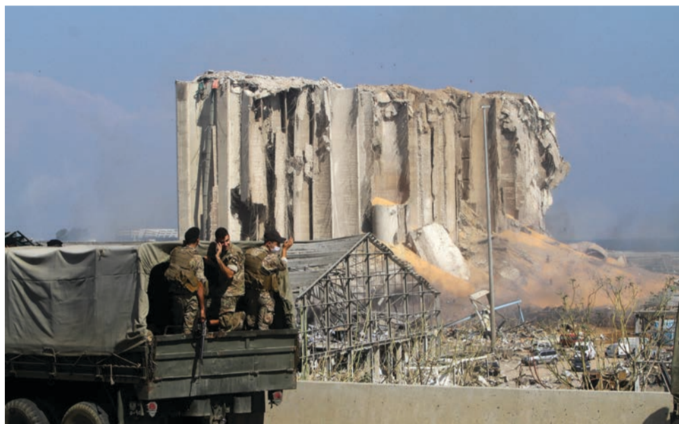
The aftermath of a massive explosion that rocked the Beirut port on 4 August 2020. The blast, the cause of which is still under investigation, was apparently felt as far away as Cyprus. | Photo: Flash90
